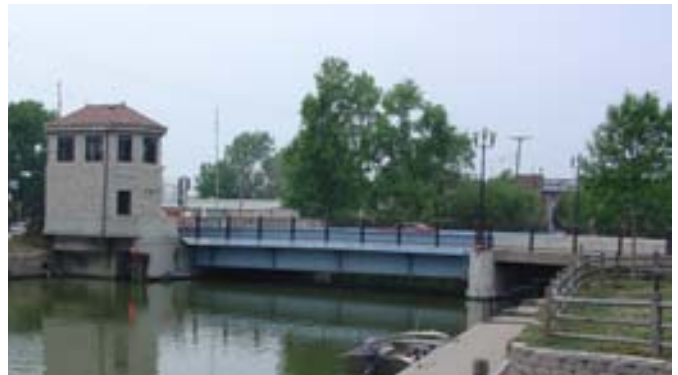
Tayco Street Bridge in Menasha may be ready for remote operation in May 2007.
