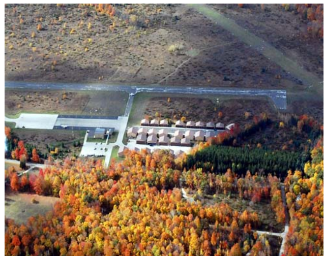
Airport Hangar area
